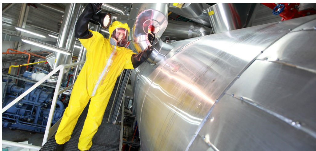
FIGURE 24: Ammonia can be safely used on board ships using established materials and safety processes
